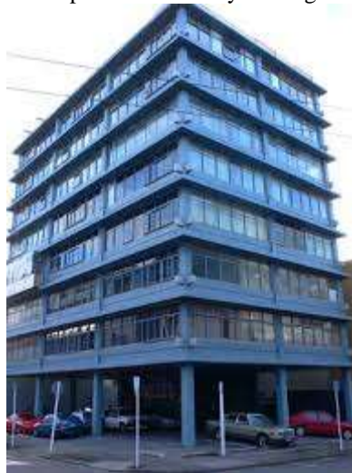
Fig 1.2 Example of soft storey at different levels
